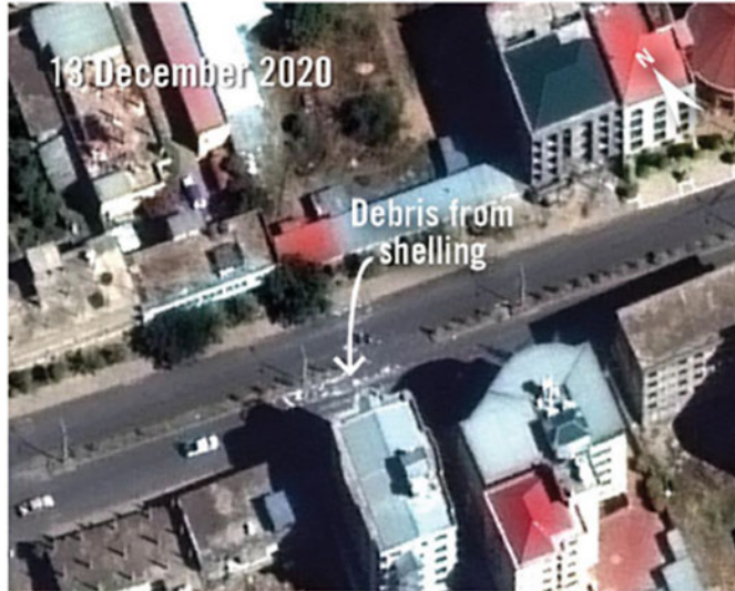
Debris from shelling is visible in front of the Brama Hotel, on Asim's old main road, in this satellite imagery from 13 December 2020. A man who had fled and who came back to the city around 25-26 November said: "After I came back to the city, I ... saw the Brama Hotel ... really damaged."
